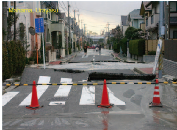
Fig. 23 Thrust of an alley in the Maihama district of Urayasu City. (Photo by Ogawa)
