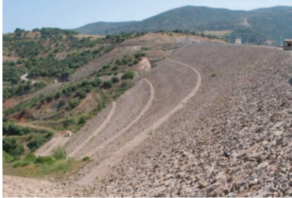
Fig. 21 Keddara dam-down-stream view
