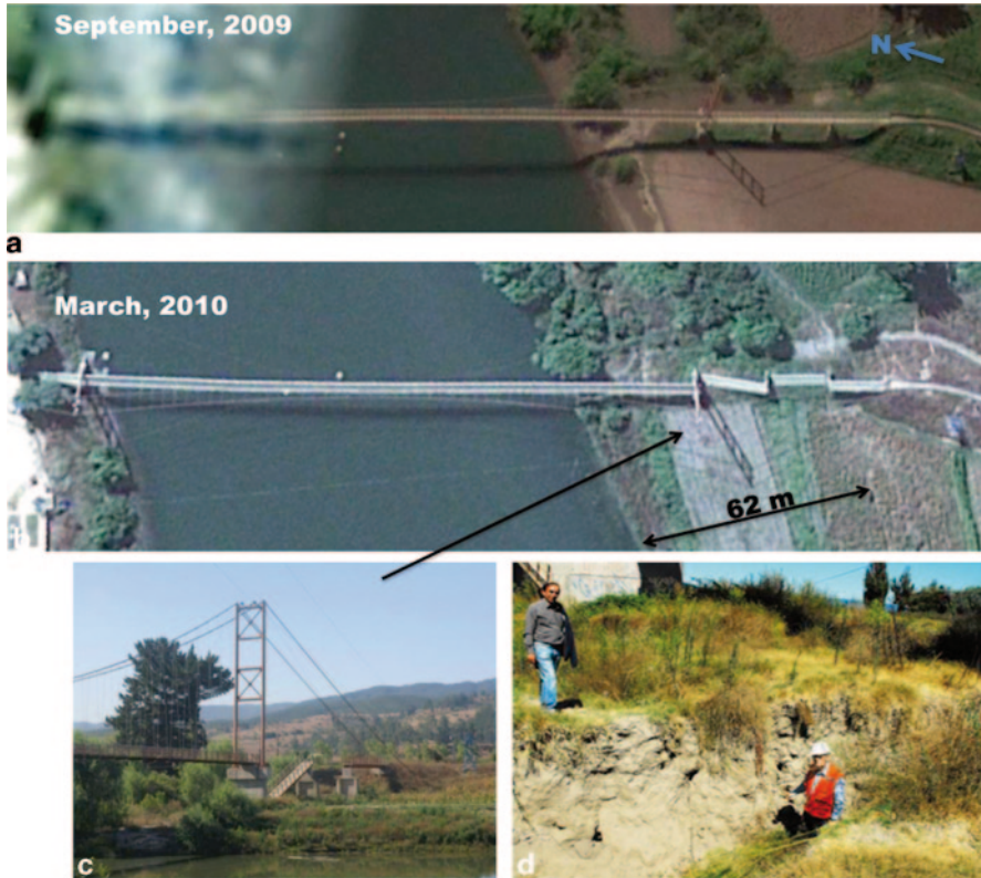
Fig. 18 Footbridge over Mataquito river. a Before and. b After earthquake (Google-Earth). c Collapse of south access. d Cracks due to lateral spreading
