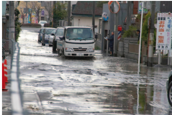
Fig. 27 Flooding of liquefied soils over the road in Sawara, Katori (from Katori city office)
