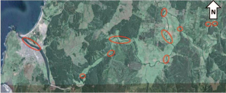
Fig. 15 Lateral spreading observed along Lebu river
