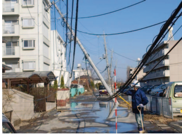
Fig. 26 Chaotic distress in the city center, Sawara, Katori (from Katori city office)
