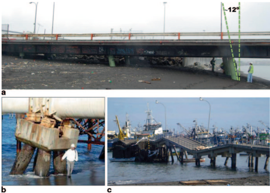
Fig. 17 Lateral spreading. a Coronel Port. b Bocamina Port and. c fishermen's Port of Coronel
