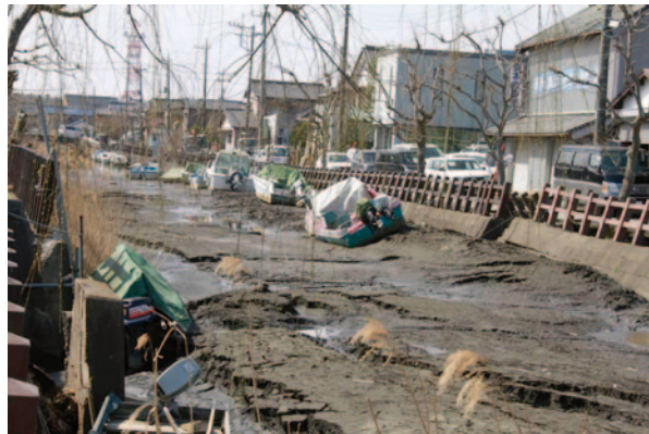
Fig. 28 Devastation in the downstream reach of the Ono River (from Katori city office)
