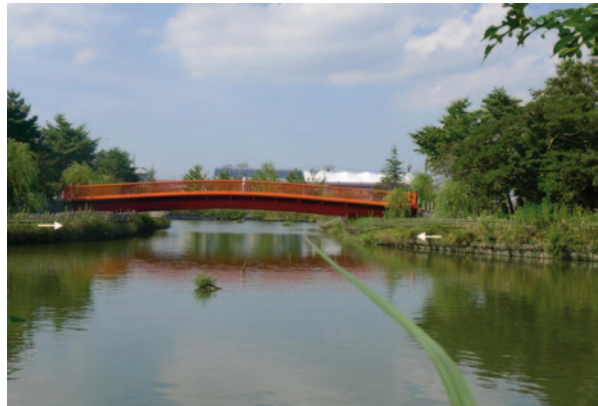
Fig. 19 General view of the bridge from the south side of the Kinrin Park at Hinode, Itako (see Fig. 13)
