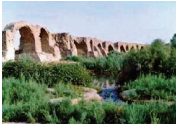
Fig. 4 Shadorvan dam-bridge in Iran. (Courtesy, ICOLD 2007)
