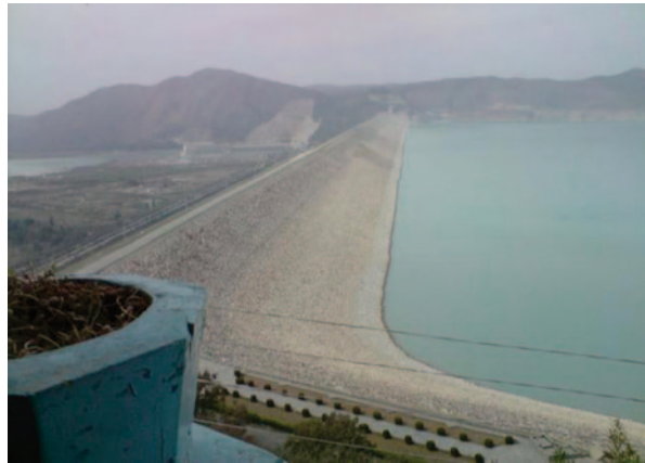
Fig. 12 Tarbela dam -general view
